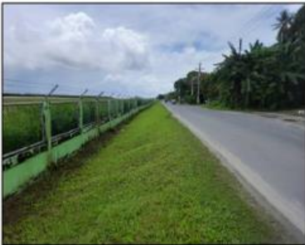
A: Airport Boundary Wall in LHS of Project Road from Ch. 0 to Ch. 2250
