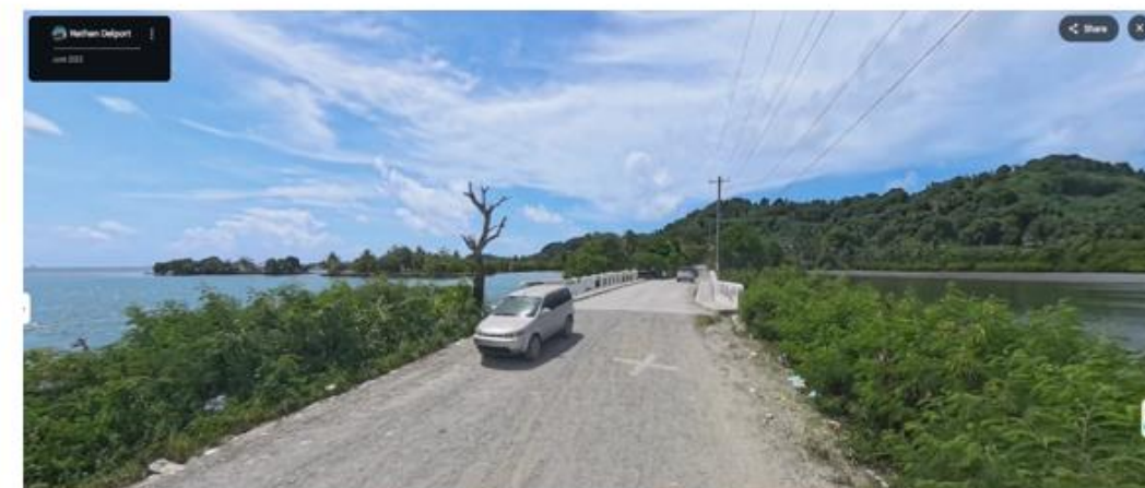
H: The end of the Airport to Pou Bay Bridge roadworks with vegetation dominated by the invasive species - Leucaena leucocephala
