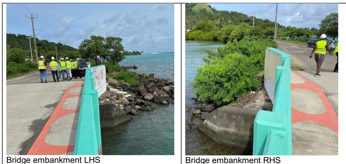
Figure 5: LHS and RHS of the bridge embankment
