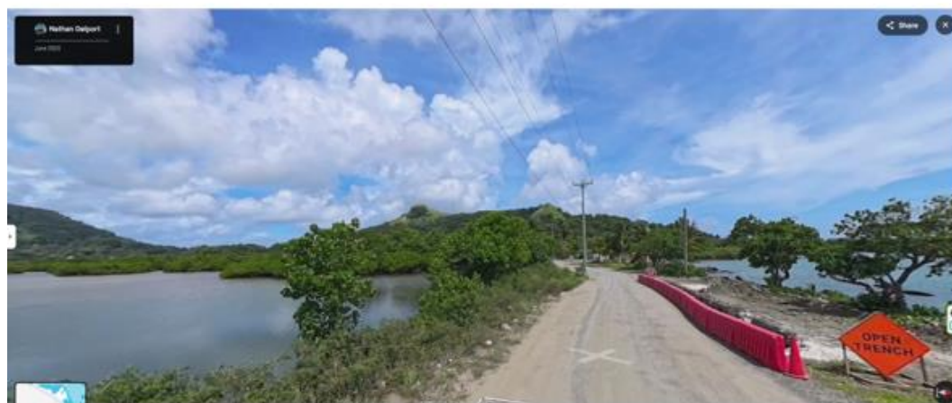
G: A small section of Pou Bay on the left and the ocean on the right. Works being undertaken for the upgrade to the Weno water supply network
