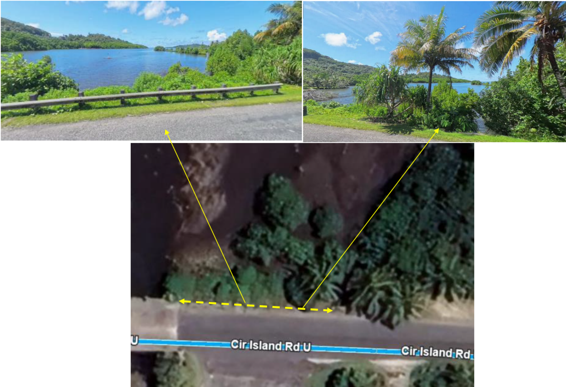
Figure 27:Vegetation overlay for embankment work along the eastern side of the Awak bridge
