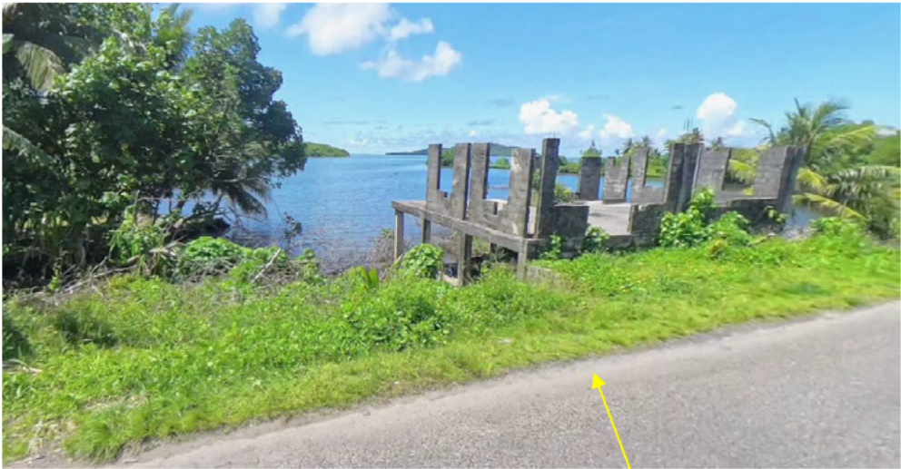
Figure 28:Vegetation overlay for embankment work along the western side of the Awak bridge
