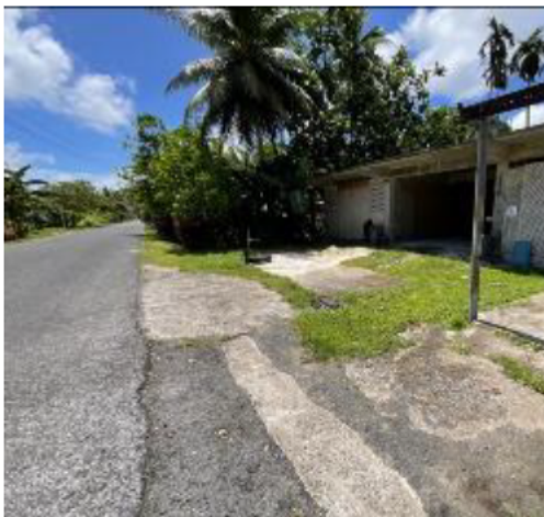
Landward side of approach road
