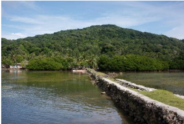
Figure 17. Example jetty in Uman
