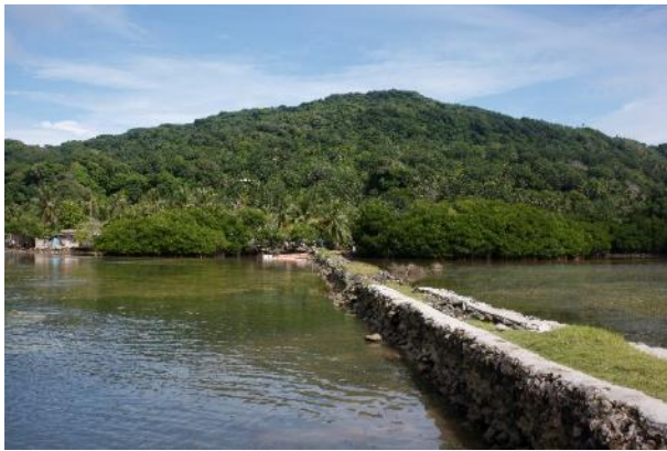
Figure 17. Example jetty in Uman
