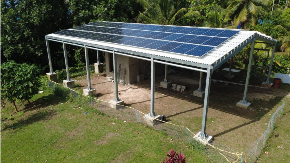
Figure 26. Example photo of a canopy with a technical building beneath (Udot Island, Chuuk)
