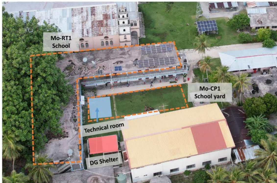
Figure 14. Aerial view of the proposed PV site for Moch
