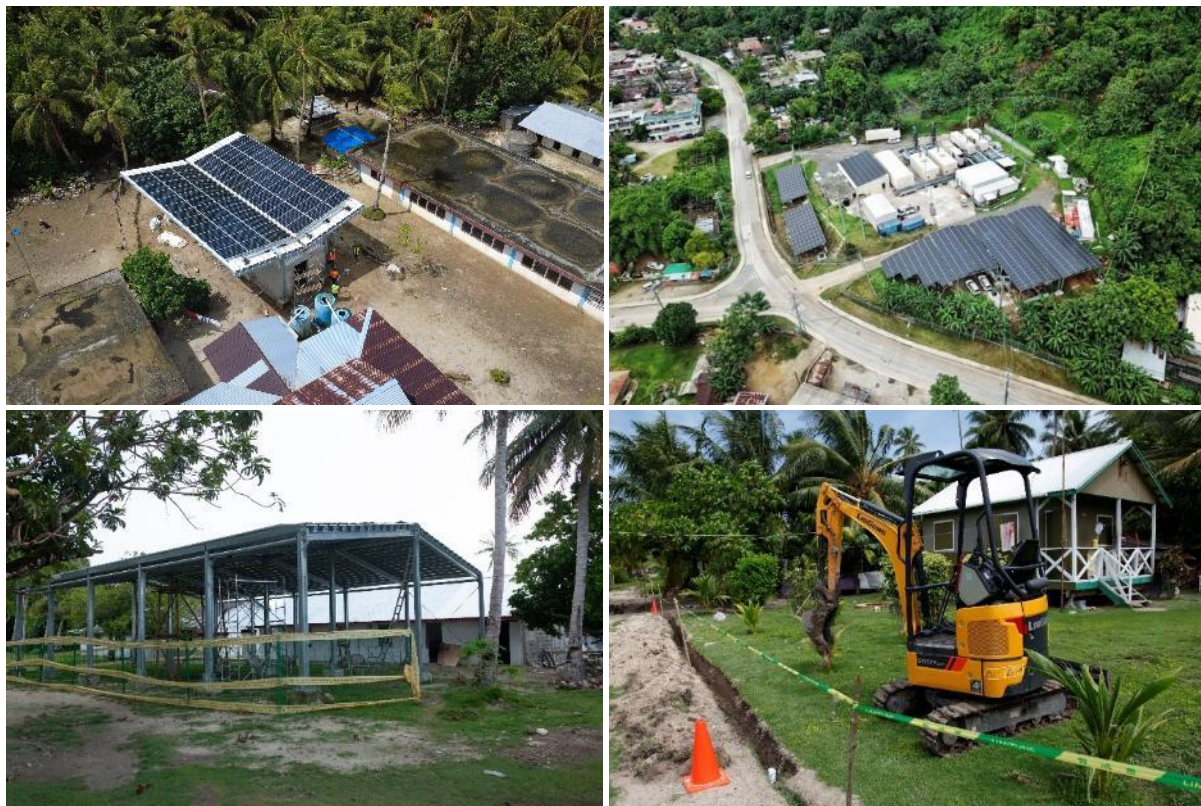
Figure 2. Pictures of energy projects in Chuuk
