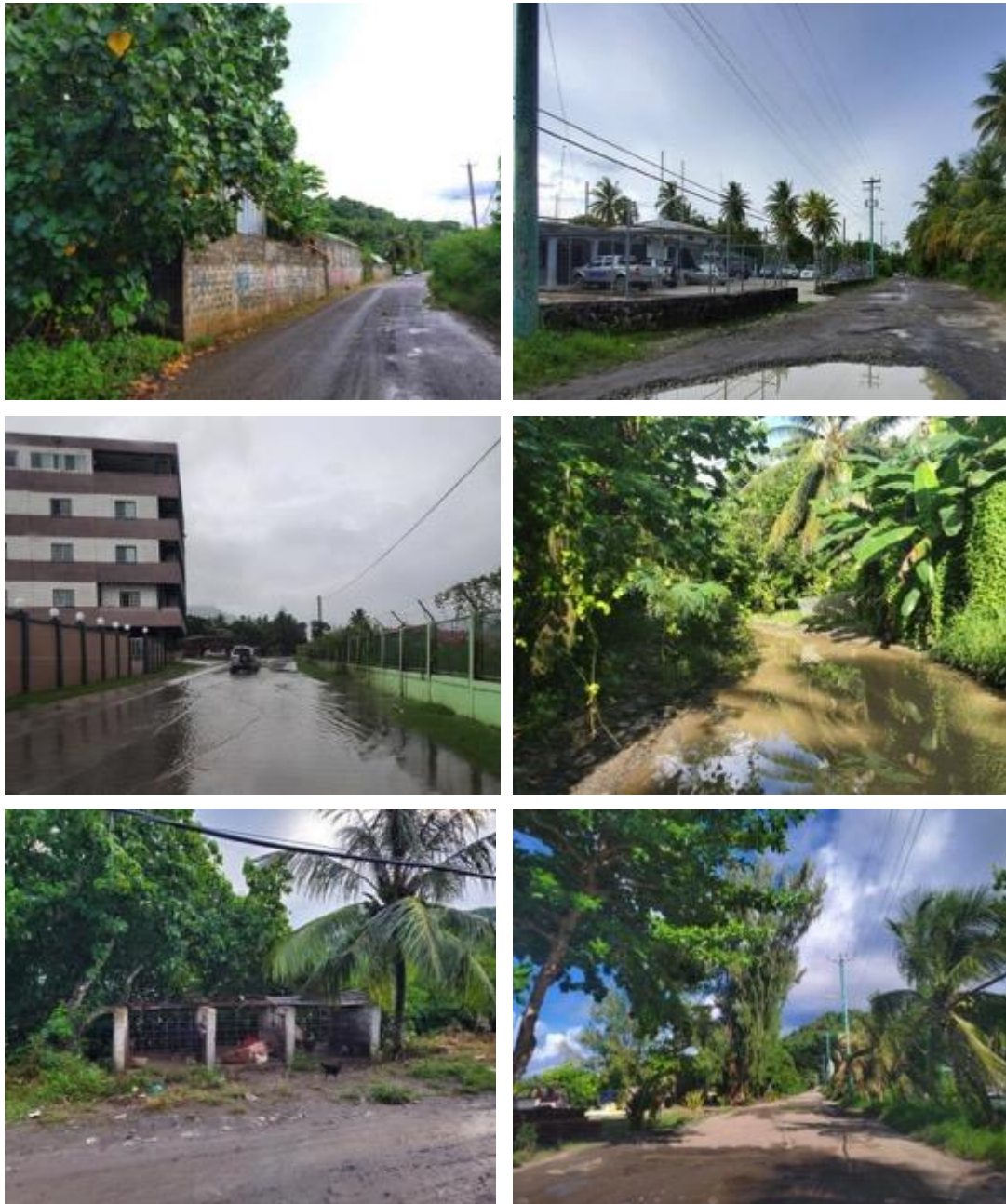
Figure 2-6: Images of Chuuk showing examples of assets and sensitive receptors identified during the road corridor on Chuuk inspection including walls and private fences (top and middle left and right), pig pen (bottom left) and power poles (bottom right).
